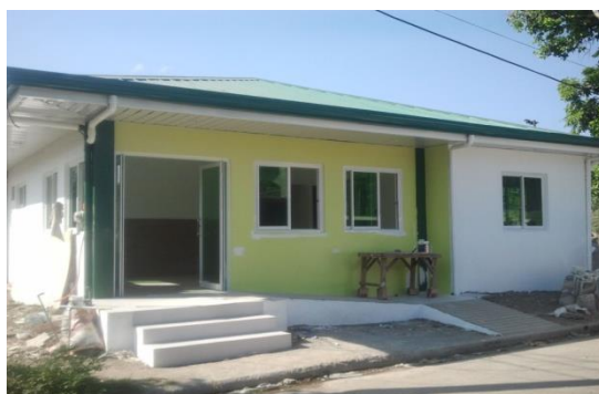
Figure 37. Patria BEMONC Facility
