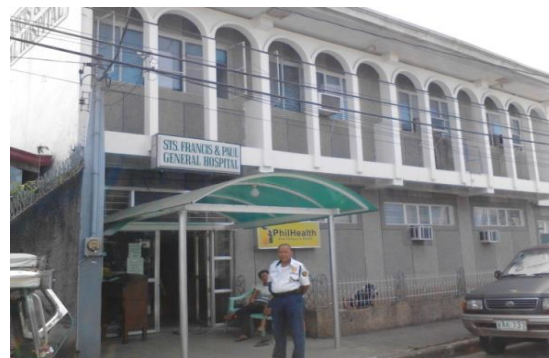
Figure 25. STS. Francis & Paul Hospital
